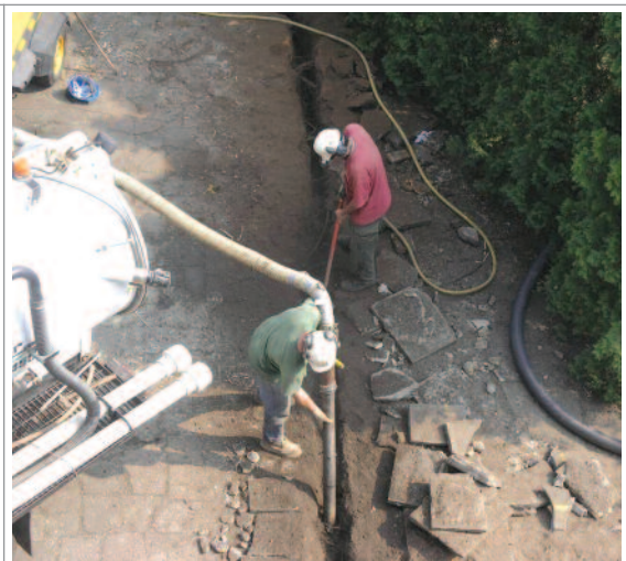
Excavating around tree roots using an air spade to avoid damage.
