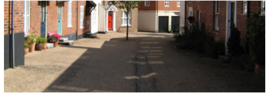
1 Shared residential Lane, bound gravel on tarmac, not delineation, central drainage
