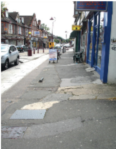
Figure 16b: Radlett District Centre | Negative features from Conservation Area Appraisal report Zone1: Patched tarmac, concrete in front of shops (a), over-use of bollards (b)
